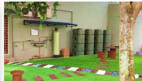
Installation of Rainwater Harvesting System
