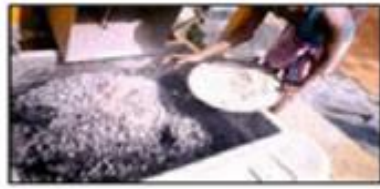
Shredded polymer waste is added to heated stone aggregate for 30-40 sec and mixed for uniform coating
