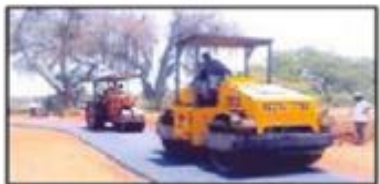
The mix known as waste plastic-aggregate bitumen mix can be used for road laying at 110-120°
